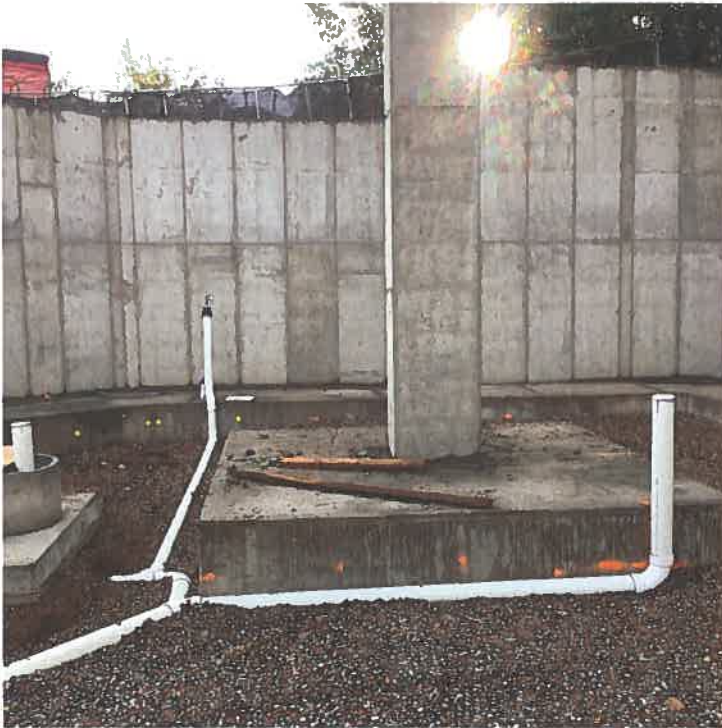
UNDERGROUND PLUMBING - 6" AND 4" LINES
