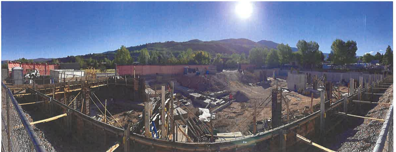
OVERVIEW OF THE SITE, SOUTH VIEW
