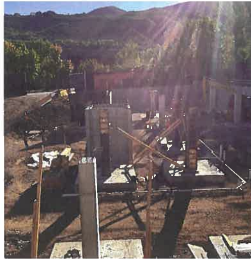
COLUMNS AT FRONT OF ELEVATOR PADS
