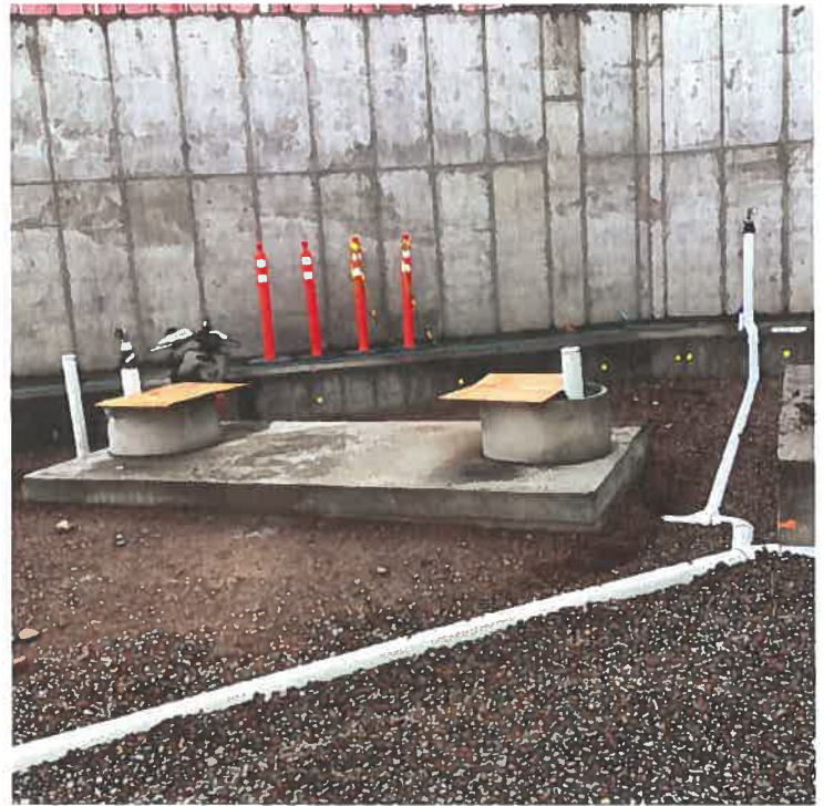
UNDERGROUND PLUMBING - 6" AND 4" LINES
